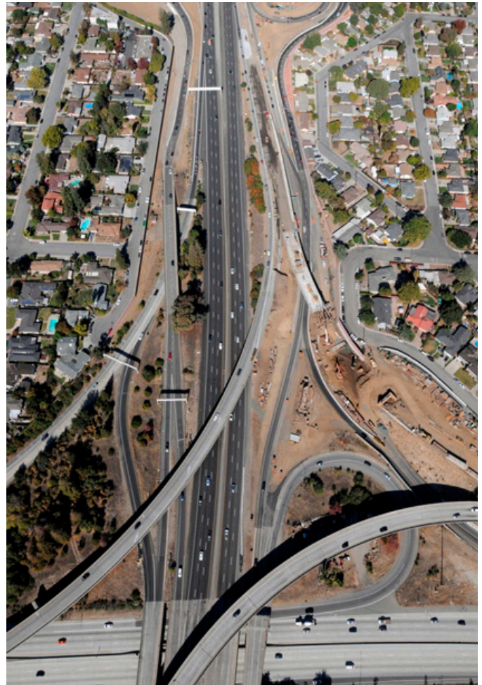
Aerial View of the I-280/I-880/Stevens Creek Boulevard Improvements Project
